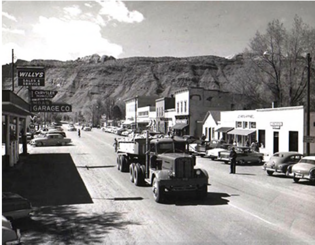
Ore truck headed north on Main Street. Mid-1950s
